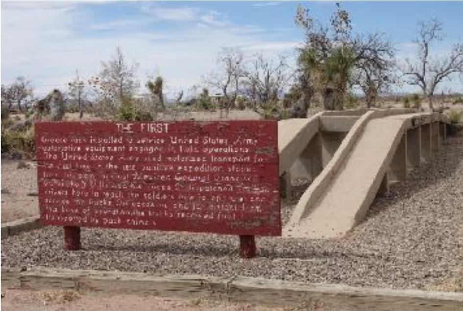
*The first grease rack — made of concrete.*
