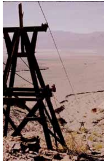
Remnants of the Keane Wonder Mine high above the valley
