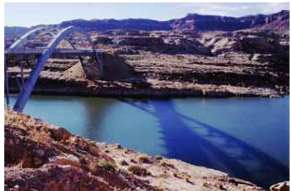
bridge carrying Utah 95 over the Colorado River at Hite Marina
